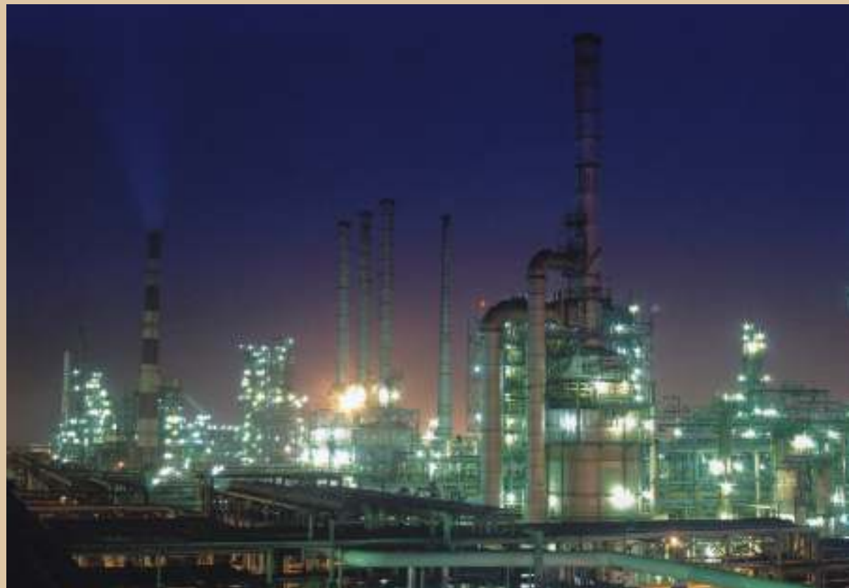
MRPL: Refinery Units.
