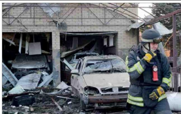
A rescue worker near a house damaged after a Russian attack on Zaporizhzhia, Friday
