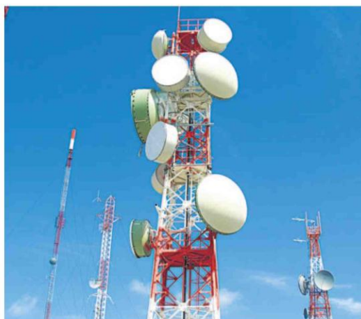
State-level restrictions on diesel sales, triggered by the conflict in West Asia, are disrupting fuel access for telecom towers despite the sector's critical tag.
