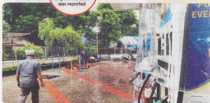
A worker pumps out contaminated fuel from the affected tank. PIC/SARTHAK MEHTA
