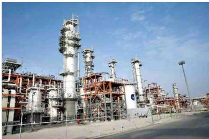
REPRESENTATIONAL IMAGE OF THE PETROCHEMICAL PLANT
