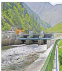
PSPs use water's kinetic energy to create a stable power supply.
