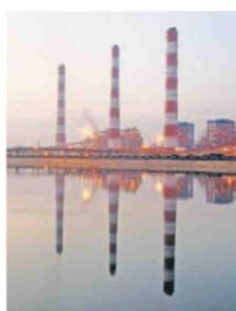
NTPC's first methanol plant likely to be completed by July.
