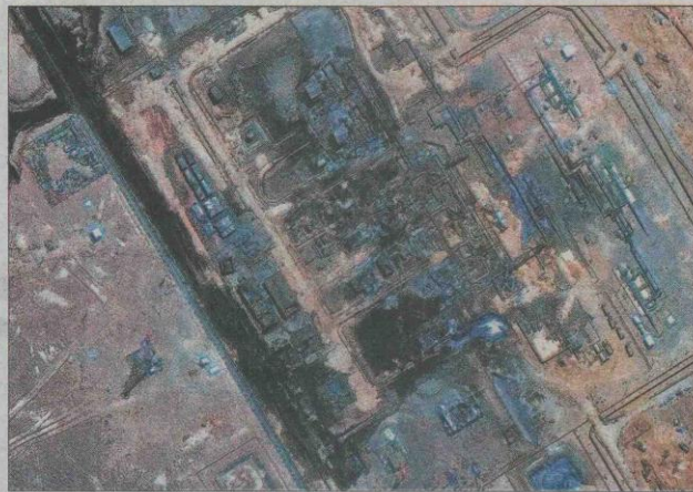
A pumping station along the general route of Saudi Arabia's East-West pipeline (Petroline) in al-Mesabaah, southeast of Medina, on Sunday, following an attack and resulting fires.
