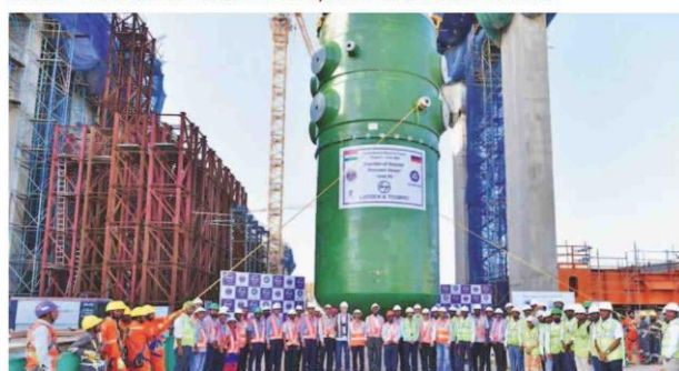
Unit-5 of Kudankulam Nuclear Power Project, in Tamil Nadu
