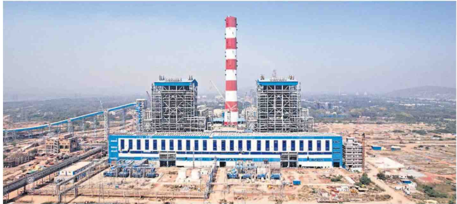
The first ultra-supercritical unit of the 2×800 MW Telangana Super Thermal Power Project of NTPC-Ramagundam reached its full capacity performance by producing 801.6 MW on Sunday night.
