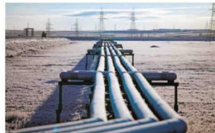
The Centre ordered a streamlined and time-bound framework for laying and expanding PNG pipelines. BLOOMBERG
