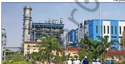
SWITCHED ON: Yelahanka power station, which had remained shut for over four months, resumed operations Monday
