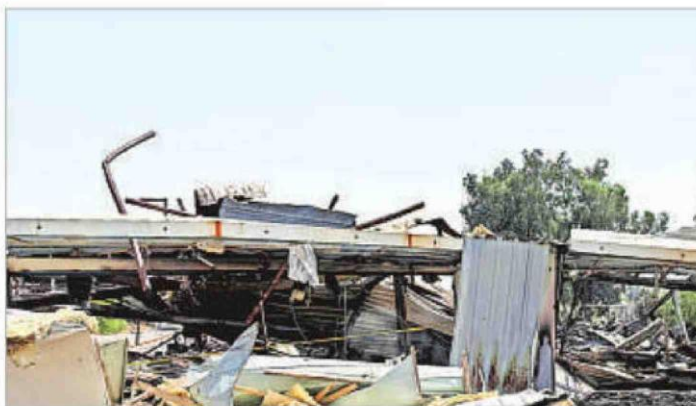
Damage at a site belonging to Iraq's Popular Mobilisation Forces (PMF) following airstrikes that the PMF said were carried out by US and Saudi forces on Wednesday
