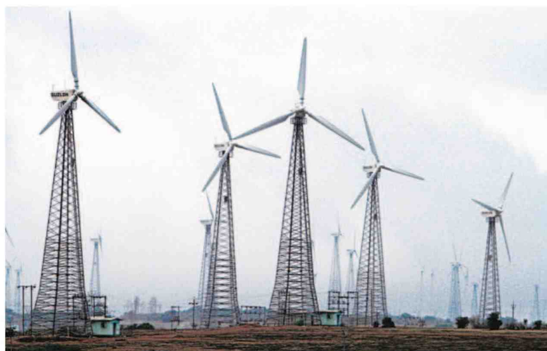
Sembcorp's installed and under-development renewables portfolio in India is at 3GW
