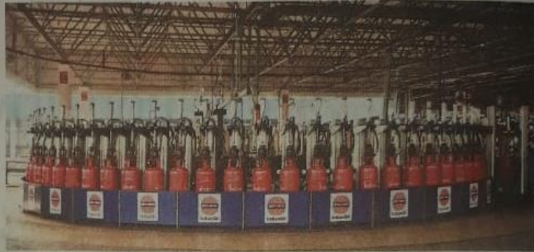
The carousel at the LPG bottling plant of Indian Oil Corporation in Cherlapally. *NAGARA GOPAL
