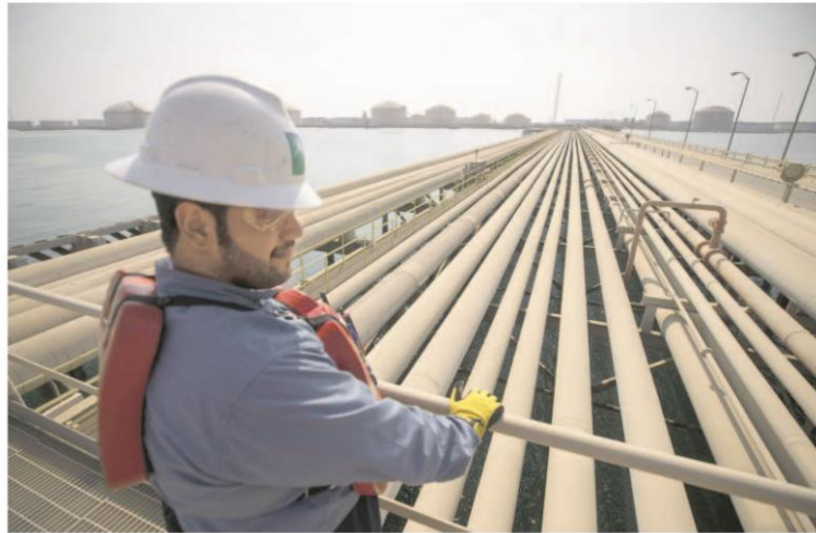
The 60 million-tonne-per-annum Ratnagiri project is a joint venture of Aramco, Adnoc, IOCL, BPCL and HPCL.
