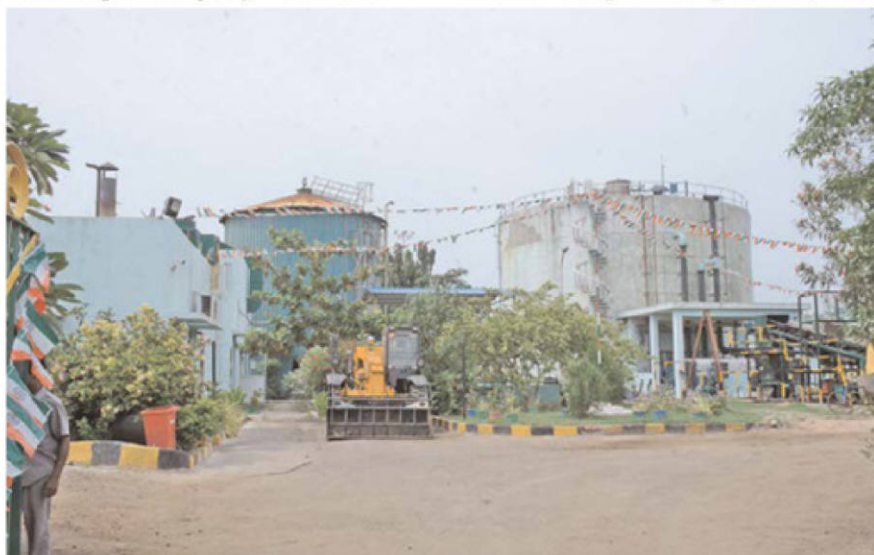
The bio-gas plant at the Koyambedu market premises.
