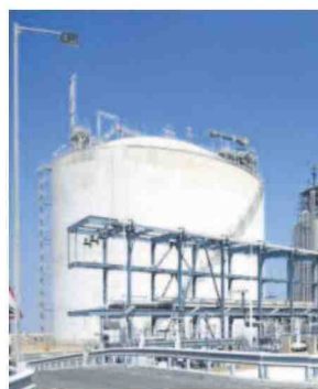
The terminal will liquify some portion of the gas flared by Iraq.
