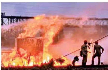
Firefighters present at the site as dark smoke, and flames billow after a massive fire broke out suddenly in a naphtha-carrying pipeline at the Haldia Refinery, on Tuesday
