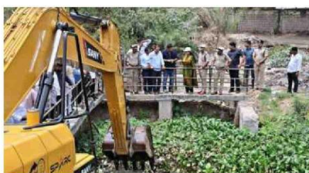
Water hyacinth being removed from Cherlapalli Lake by an earthmover as part of restoration works on Tuesday.
