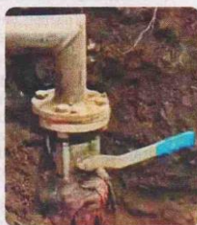
The pipeline was 40-ft. PIC/X/@EXPOSENOWNEWS
