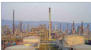
A Bharat Petroleum Corporation oil refinery in Mumbai.
