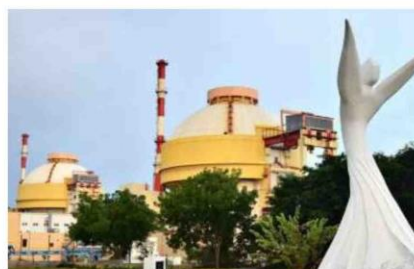
Joint effort: India's only foreign nuclear operator, Rosatom, is involved in the Kudankulam Nuclear Power Plant in Tamil Nadu.
