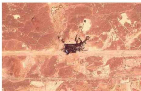
An infrastructure site after it was damaged by fire southeast of Medina along the route of Saudi Arabia's East-West pipeline. AFP
