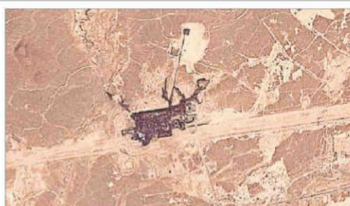
Satellite image shows damage to the East-West pipeline facility in the Hejaz Region, Saudi Arabia
