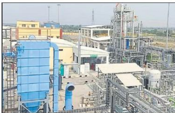
A compressed bio-gas plant.
