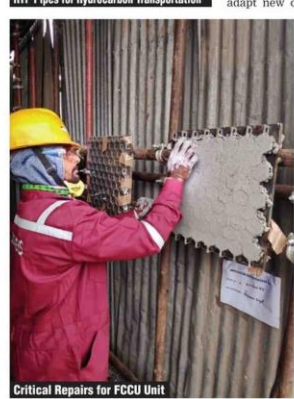
Critical Repairs for FCCU Unit
