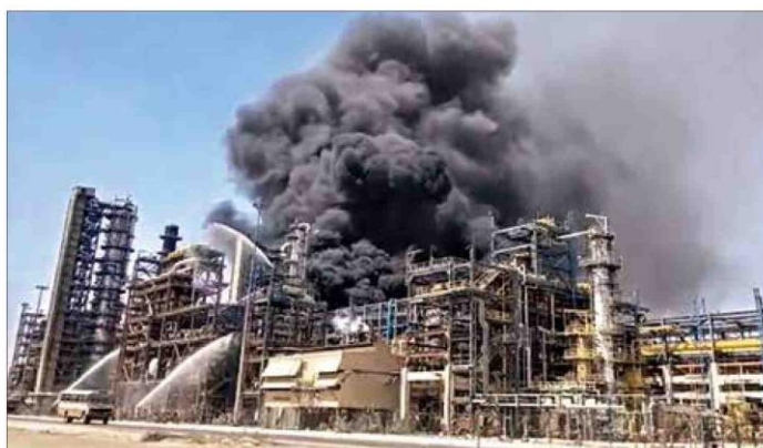
Firefighters douse a blaze after a fire broke out at the HPCL Pachpadra Refinery, in Balotra, Rajasthan, Monday PTI
