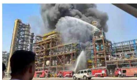
WHAT CAUSED THE BLAZE. Prima facie , it appears the leakage of hydrocarbons through one of the valves/flanges in the heat exchanger circuit caused the fire.
