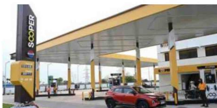
CPCL's company owned company operated (CoCo) retail outlet 'Sooper' at Manali in north Chennai BUJOY GHOSH
