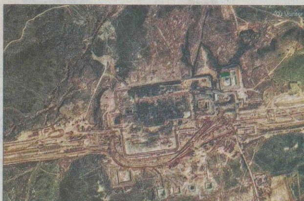
Satellite imagery shows possible construction efforts on the East-West pipeline.
