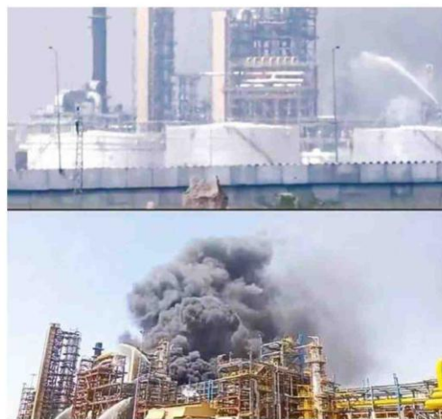
A major fire broke out at Rajasthan's Pachpadra refinery
