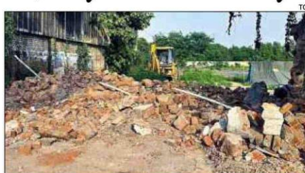
A group of 10 people, identifying themselves as AMC employees, demolished the shops in the area that falls under GIDC's jurisdiction
